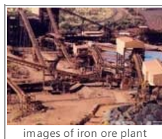
images of iron ore plant
