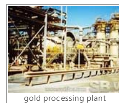
gold processing plant
