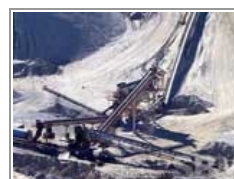
picture of double stage coal crushing plant
